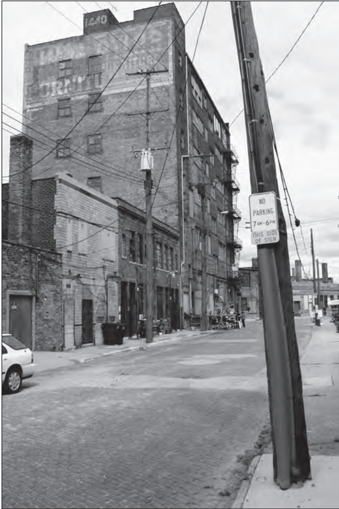
Service Street. The author's building is the third from left. [Chris Ringler]
