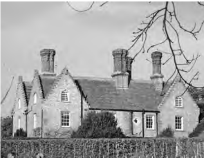
The well-appointed Victorian farmhouse built by the Cornwallises' tenant, George Neve.
