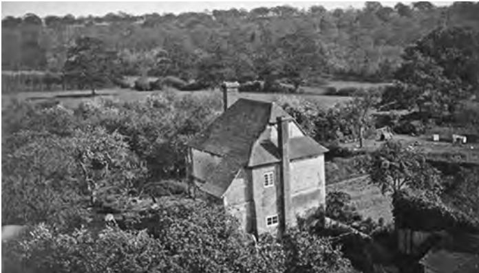
South Cottage in 1930, before the extension was added to the northern side to house the flower room and Harold's bedroom above.
